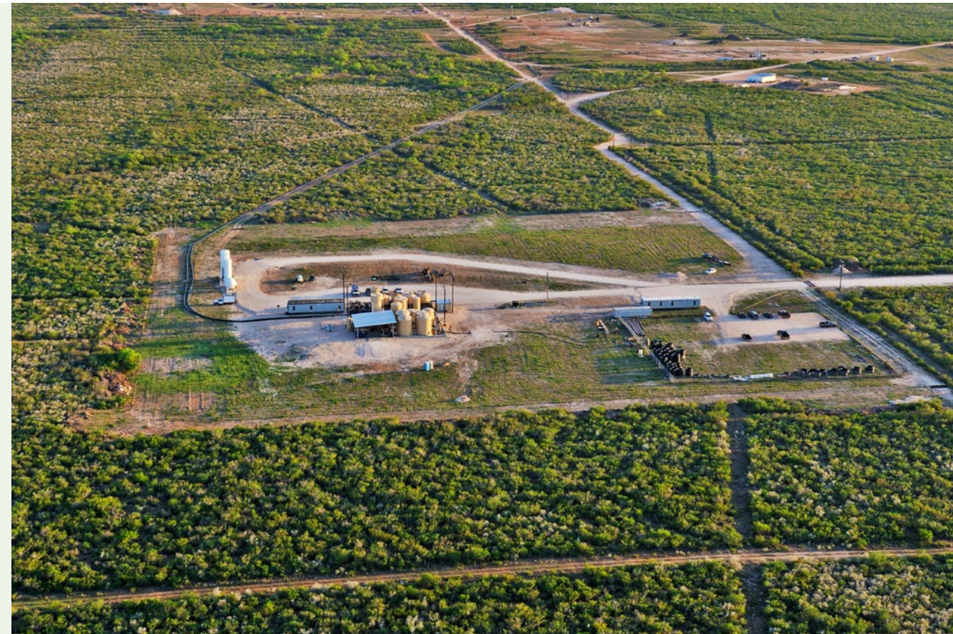
Aerial view of UEC's Palangana satellite facility
